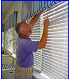
Steve repairing blinds
