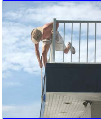
Clark scraping fascia
